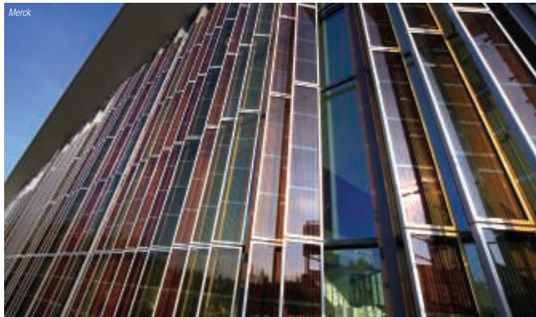
FIGURE 3. Dye-sensitized solar cells are highly efficient energy sources that can be implemented into glass units on architectural structures. Merck's work in introducing ionic liquids into DSSC systems has helped to increase the possible service lifetime of these devices
